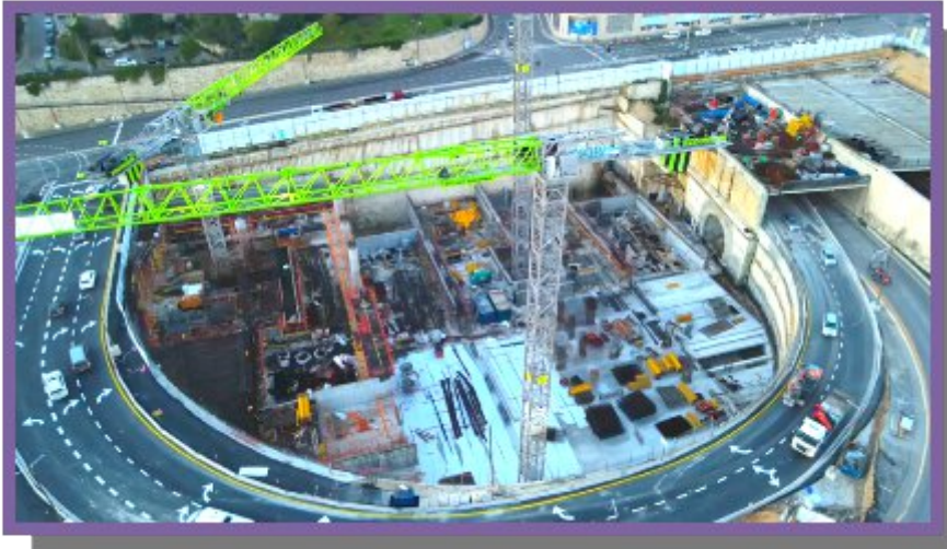
Figure 10: Jerusalem LL - Construction of the LRT Park & Ride Facility
